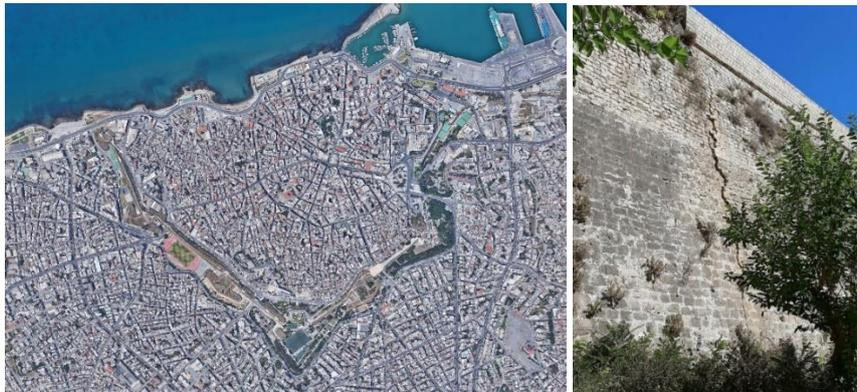
**Figure 1. (a) A satellite image of the Heraklion City bastion fortification system (Google Earth) (b) The three (3) construction phases of the line-segment Bembo-Saint Francis can be easily distinguished. A vertical crack is also visible**
